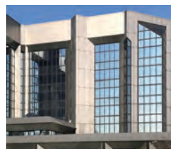
Fujitsu General Commercial Air Conditioning Italia S.p.A. (Włochy)
