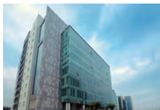
ABS Aircon Engineers Private Ltd. (Indie)
